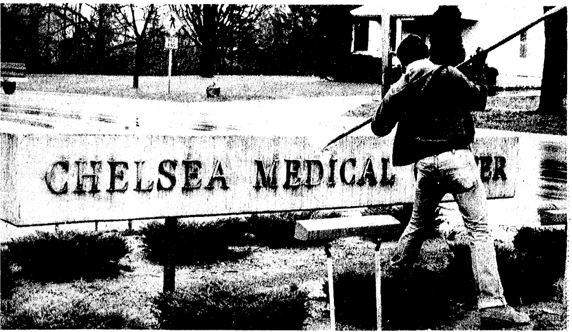
OLD SIGN REMOVED: It was a classic, graceful sign that graced the entrance to Chelsea Hospital, but, unfortunately, difficult to see at night. Last week, a hospital worker began slowly chipping away at the stone block to make way for a new, more visible sign.
